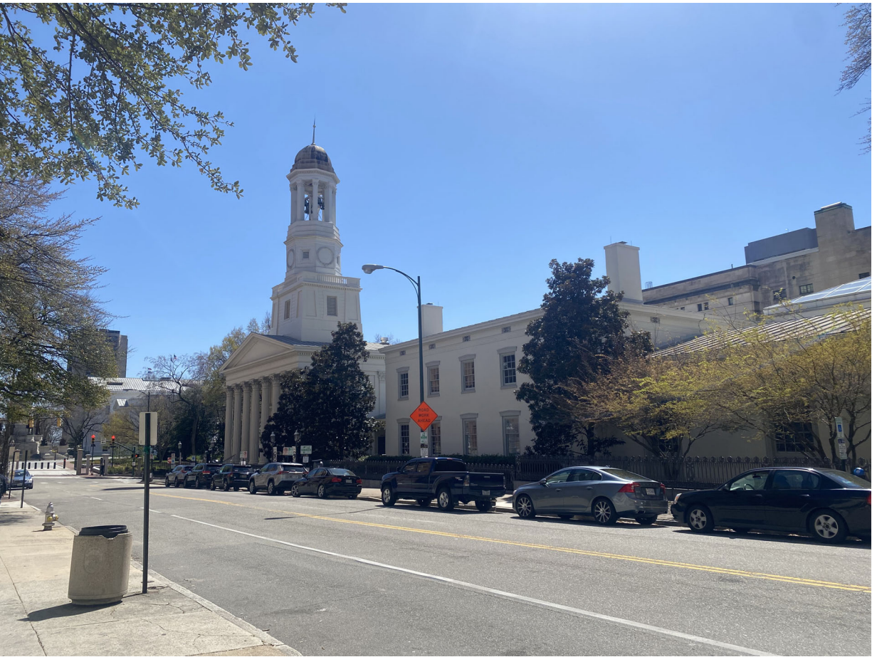
17. View from Grace Street - limited visibility from one location
