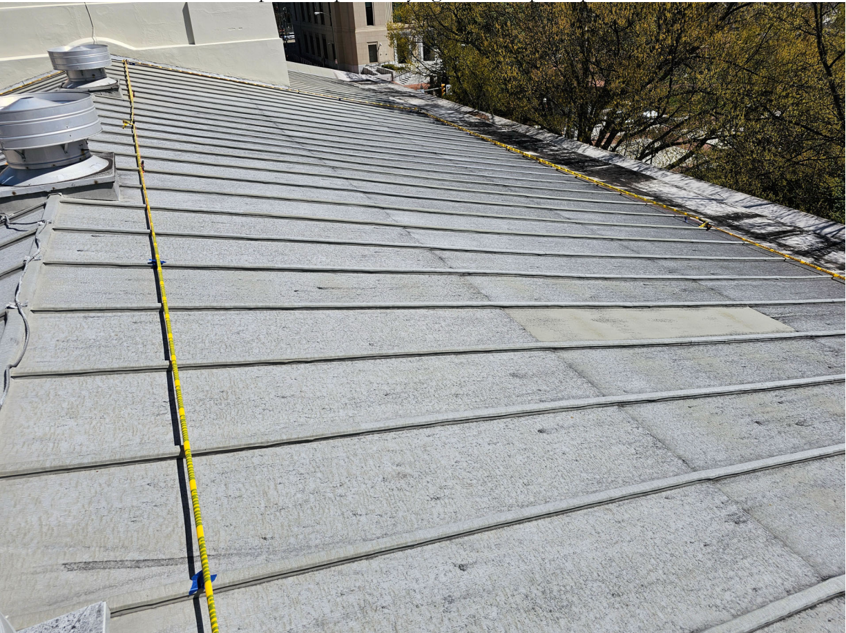
2. Rooftop mockup identifying extent of panel placement
