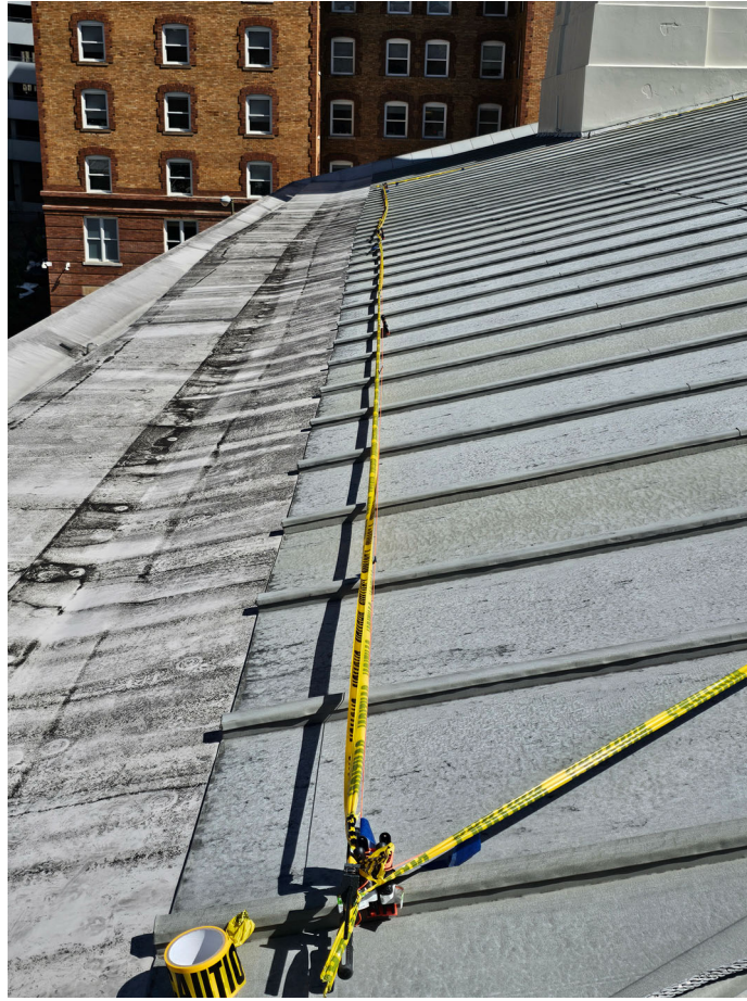
1. Rooftop mockup identifying extent of panel placement
