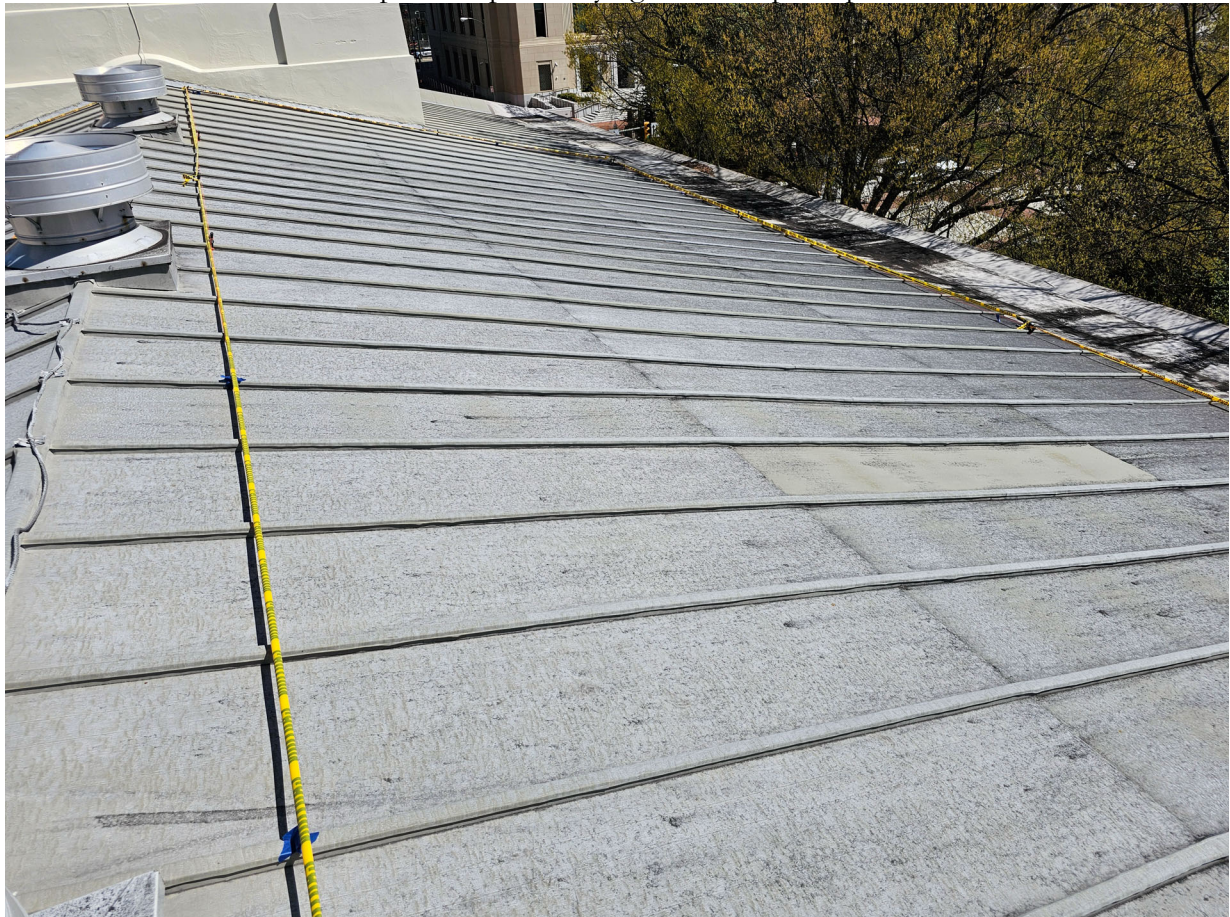
2. Rooftop mockup identifying extent of panel placement
