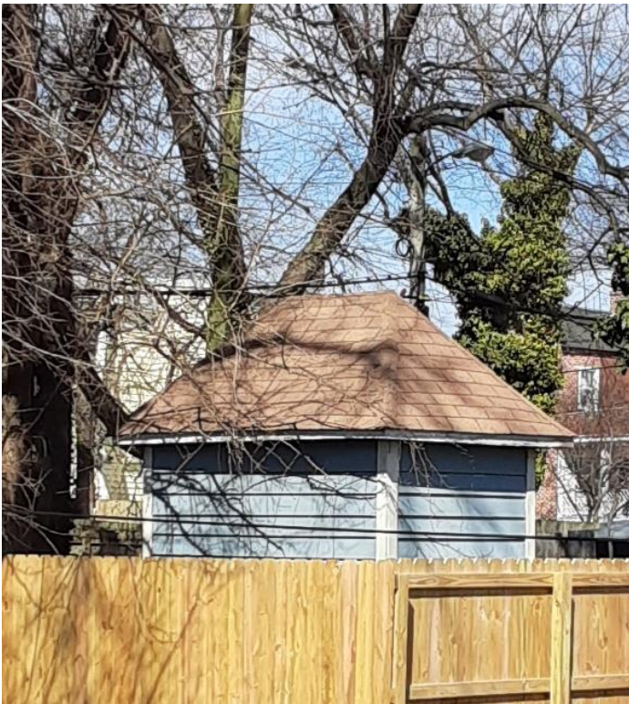
Figure 3. Existing shed on the block.
