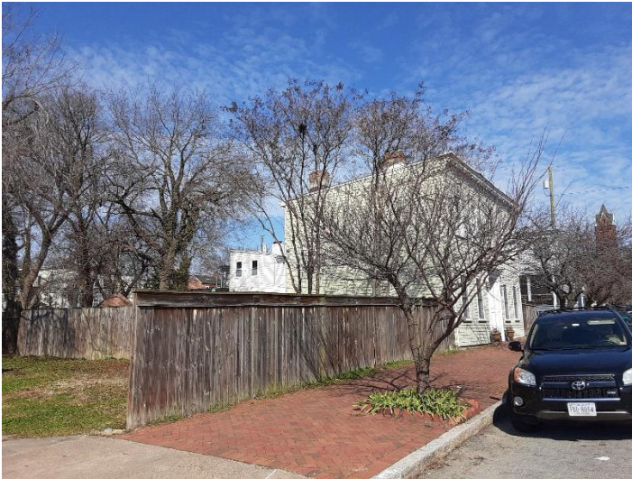
Figure 1. 608 N. 24th Street.
