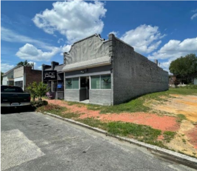
Figure 7. View of facades facing east.
