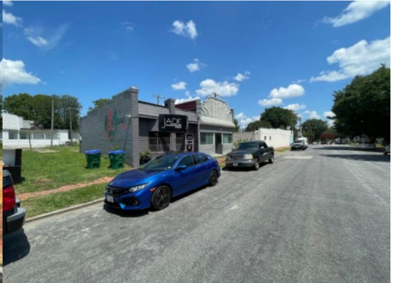
Figure 8. View of facades facing west.
