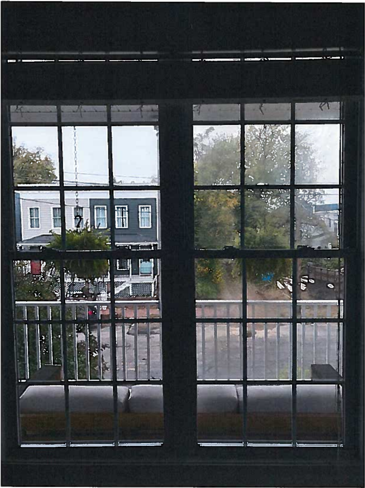
Windows 1 & 2 Full Window View
