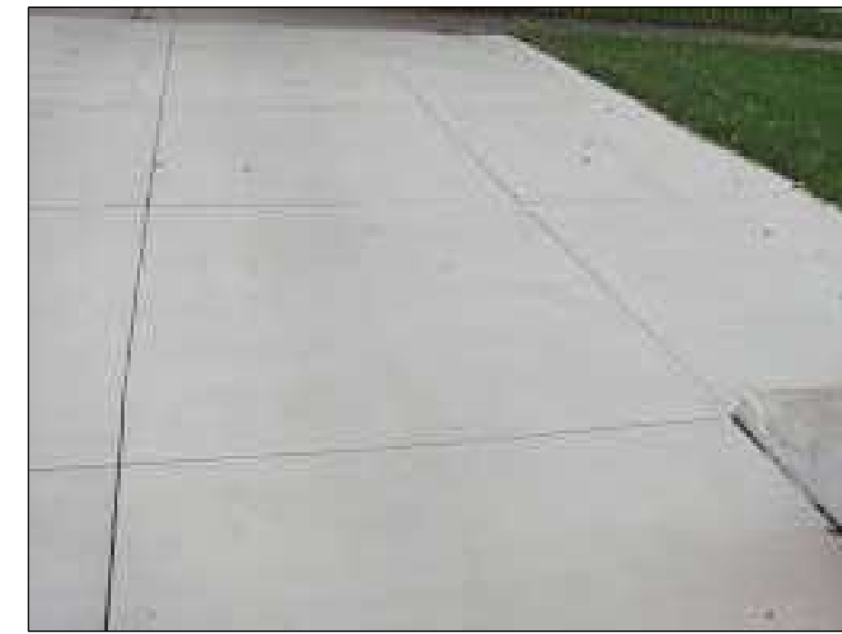
Plain Concrete @ Perimeter of Site
