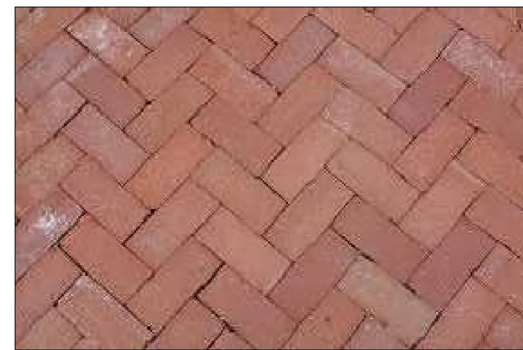
Herringbone Brick Pavers Color: Red, Reclaimed On-site brick.
