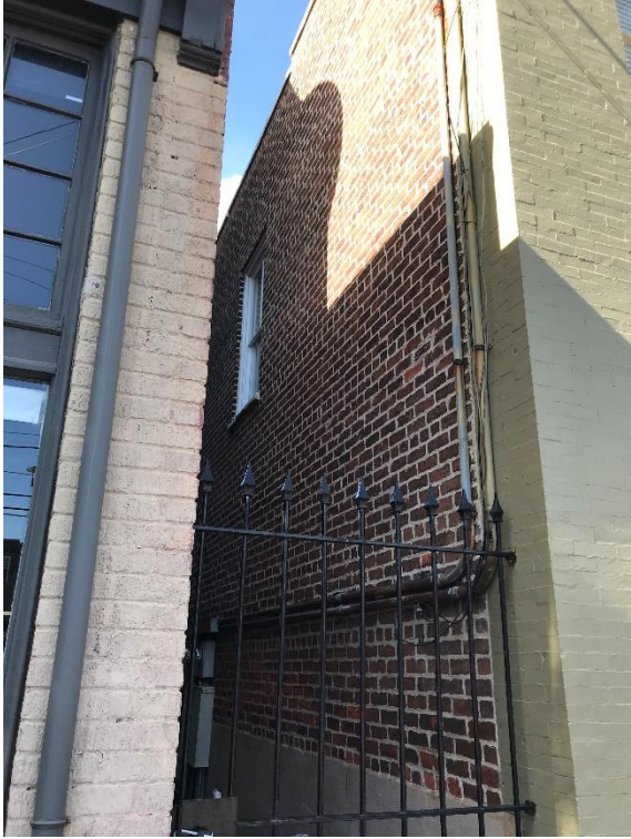
Figure 1. View of side elevation from North 26th Street
