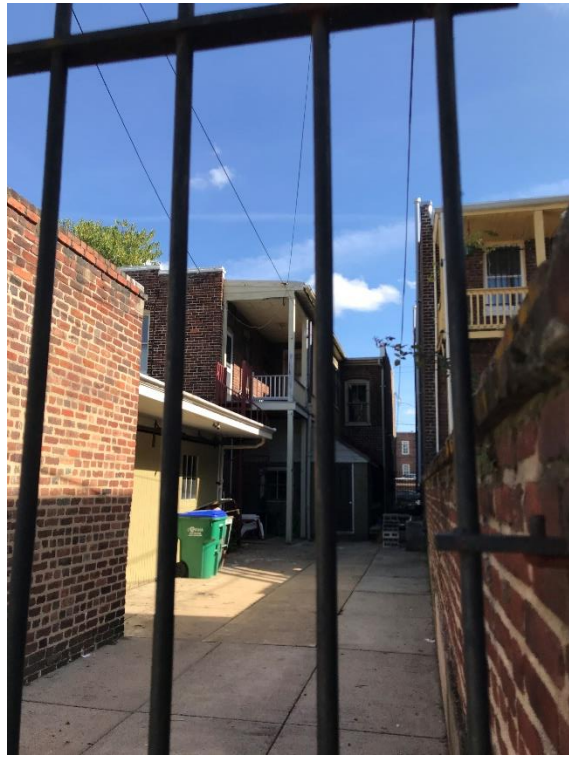
Figure 2. View of rear from alley.
