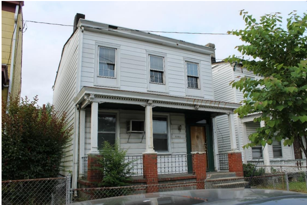
1. Façade, view to the southwest
