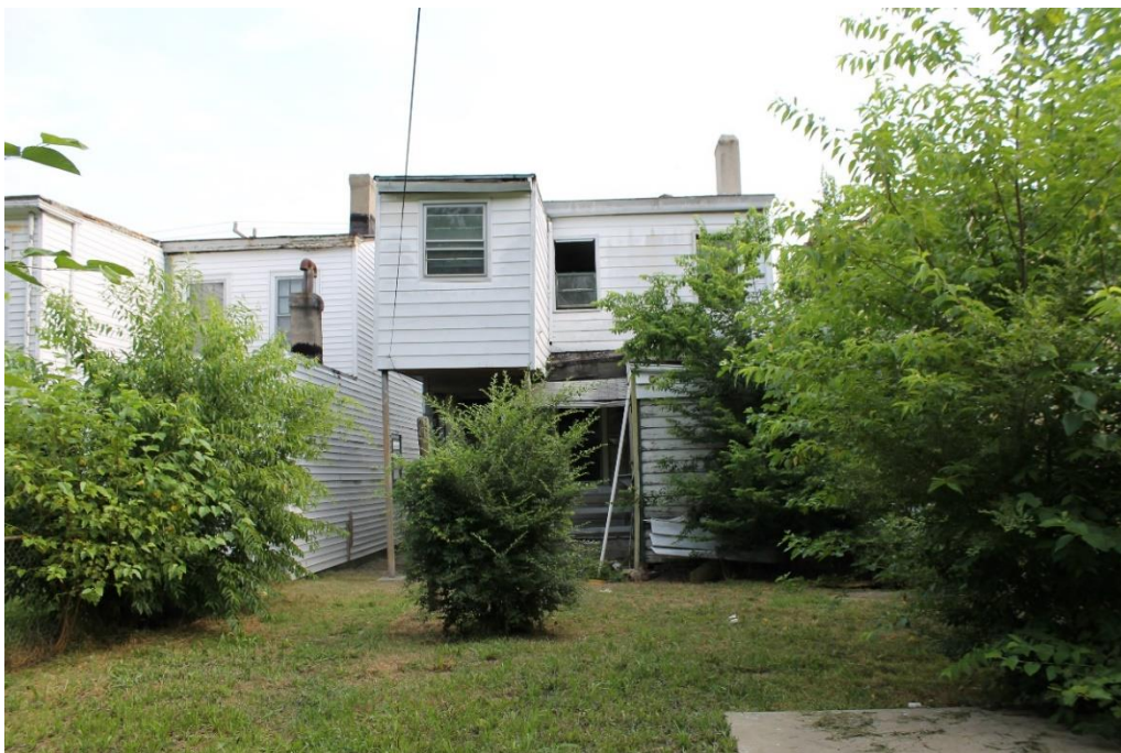
4. Rear, view to the north
