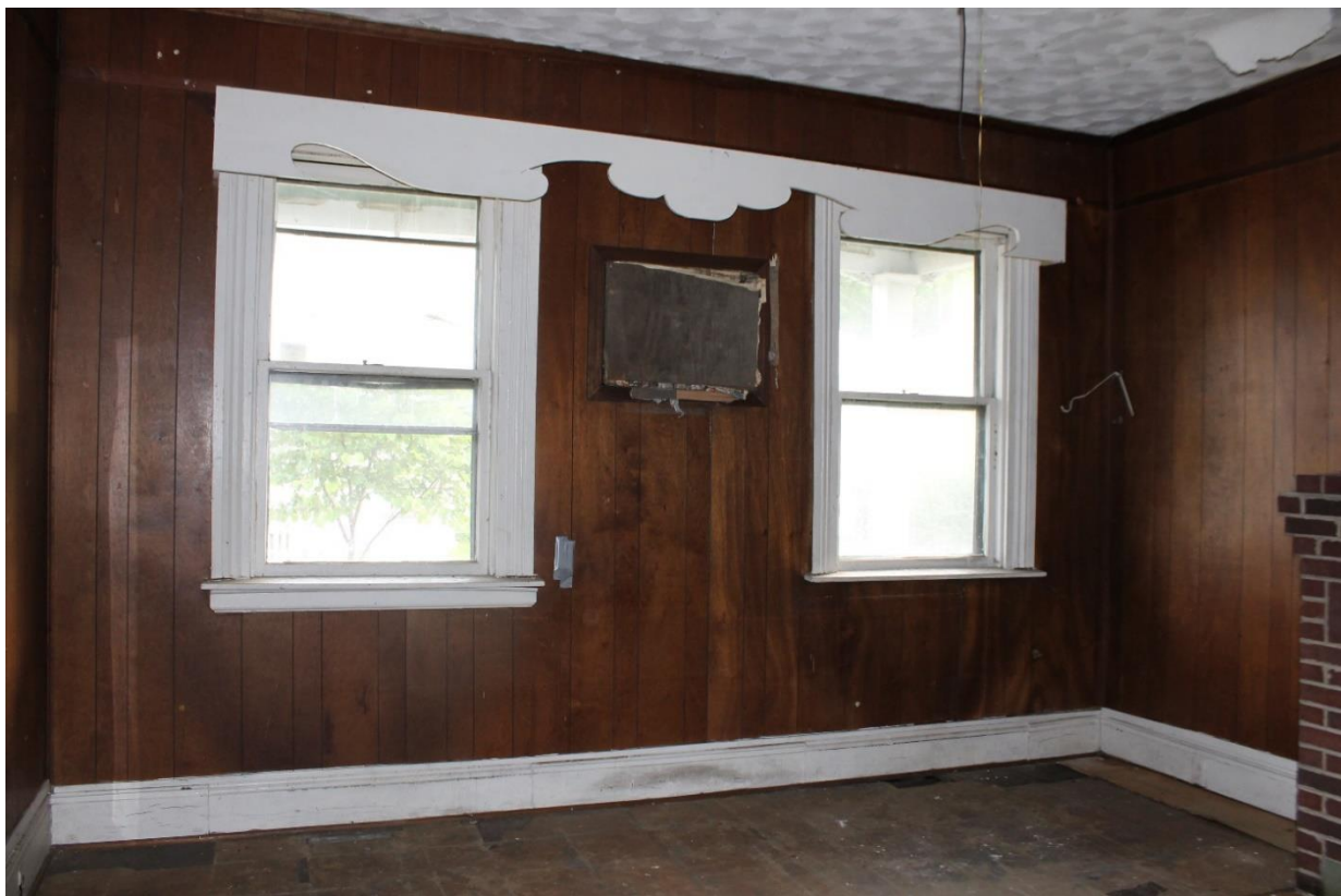
14. First floor front room looking to the front, view to the north
