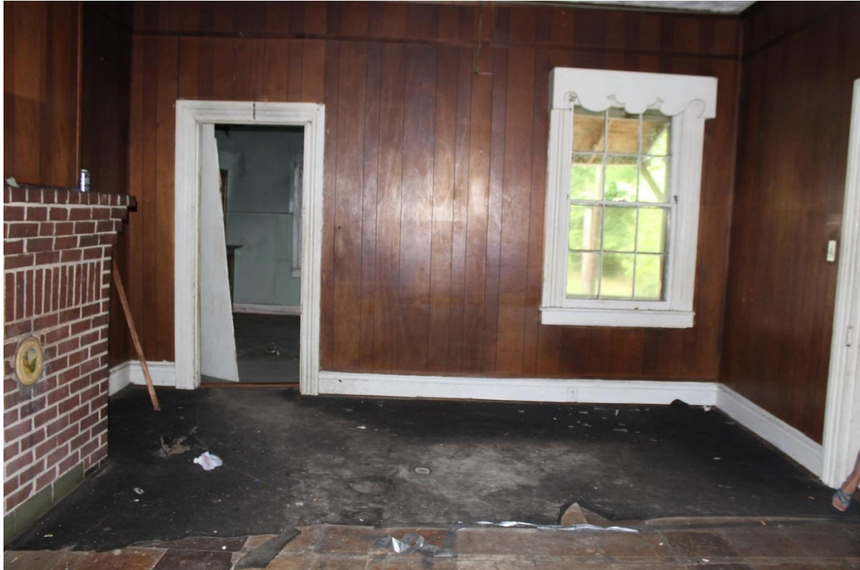
15. First floor rear room looking to the rear, view to the south
