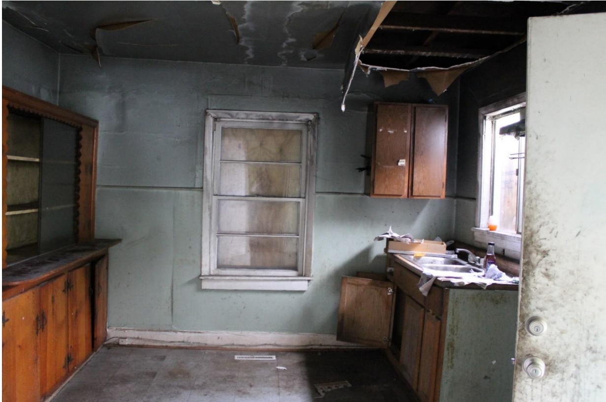
19. Kitchen looking to the rear, view to the south
