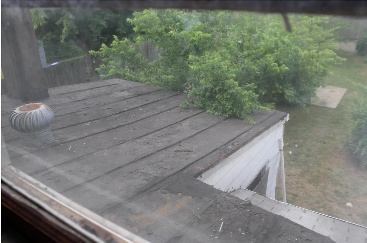
7. Roof of kitchen wing, view to the southeast
