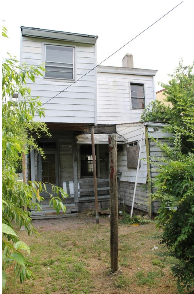
5. Rear, view to the north
