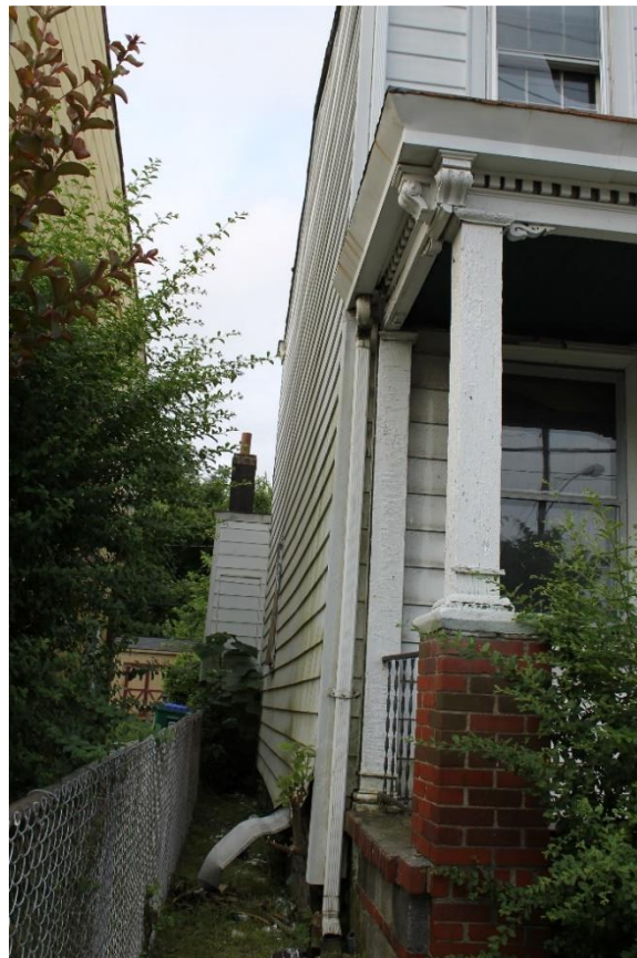
2. Eastern side and front of kitchen wing, view to the south
