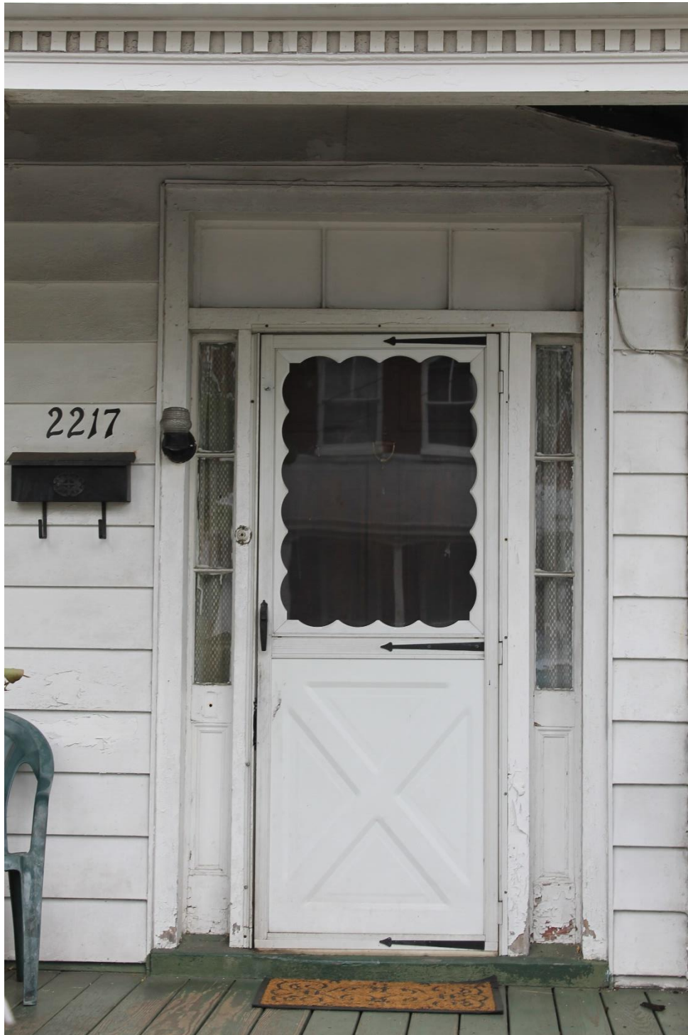
Sidelights on 2217 Venable Street to be used as model for new sidelights on 2209 Venable Street
