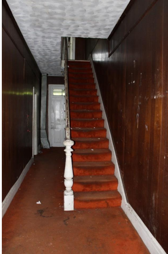
9. First floor side hall and stairs, view to the south
