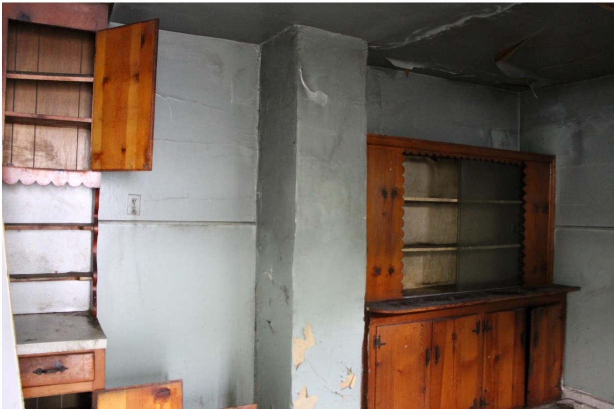
20. Kitchen, view to the southeast
