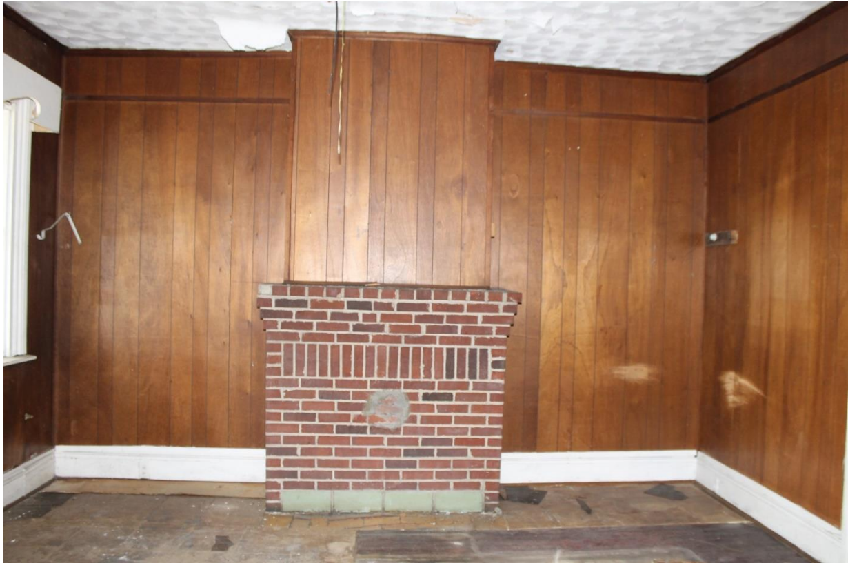
11. First floor front room, view to the east
