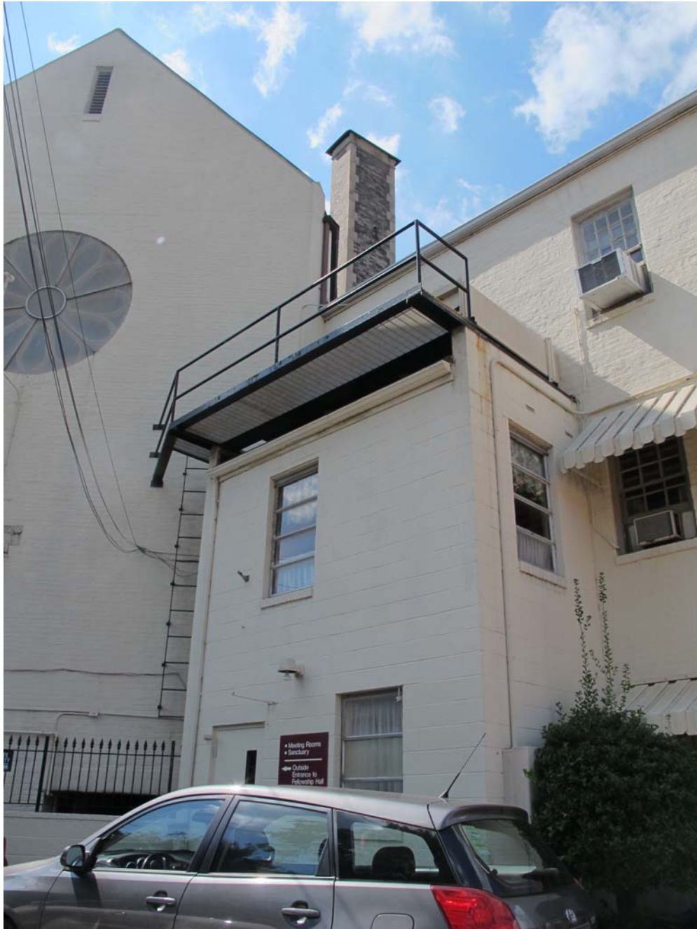
B. Rear elevation, church on L, school on R
