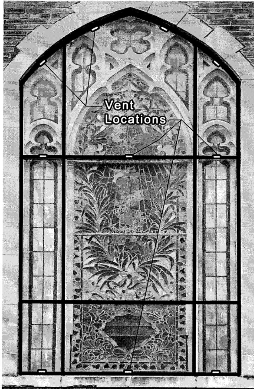
Window B - Panel configuration and support for new tempered glass option. Framing bending diagram and vent locations.
