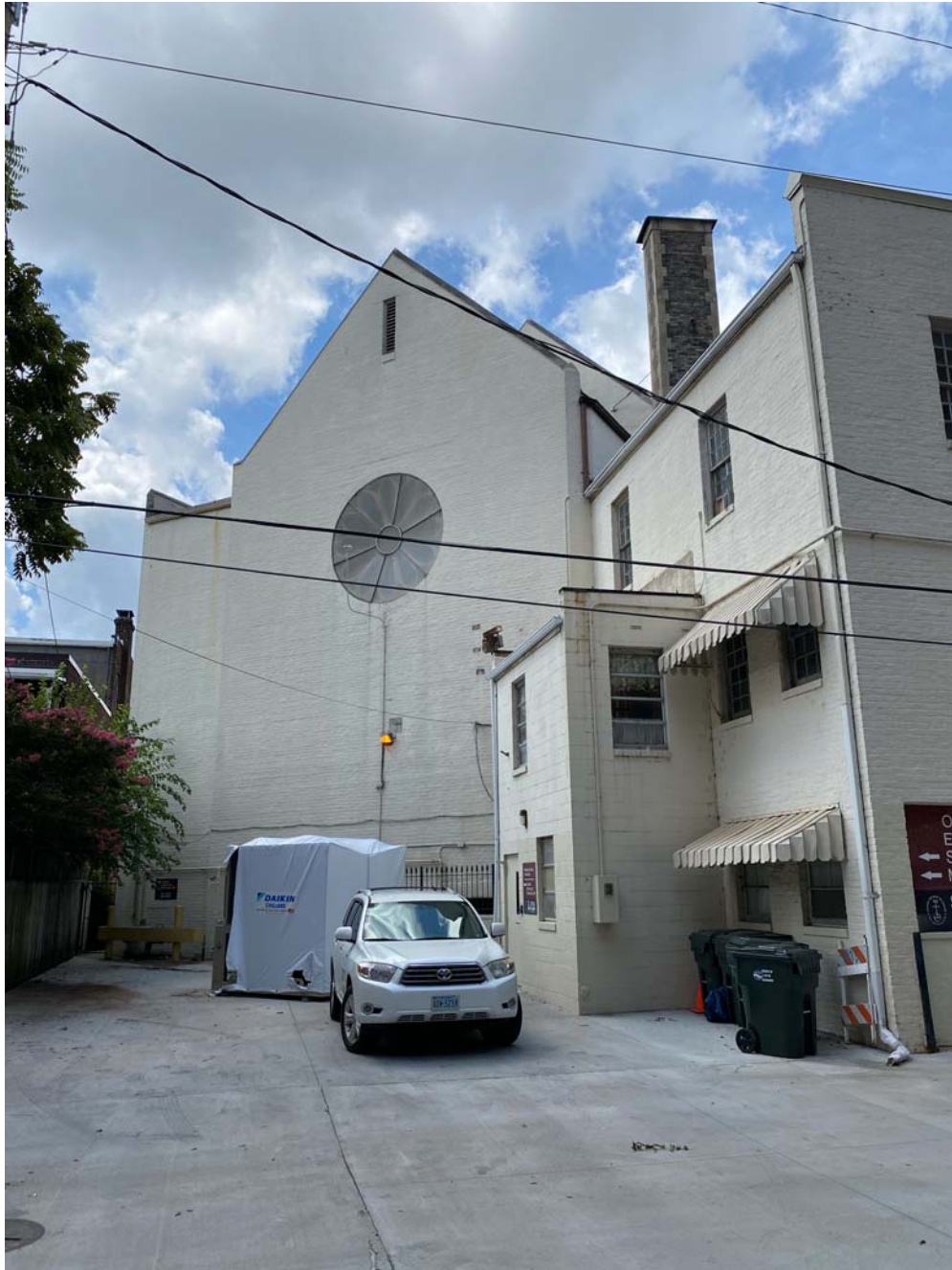
D. View of rear elevation with chiller (not final location)
