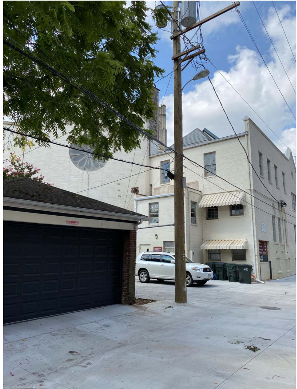
E. View west along alley
