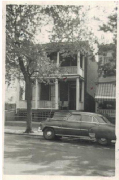
Figure 6. Original dwelling on-site. Demolished
