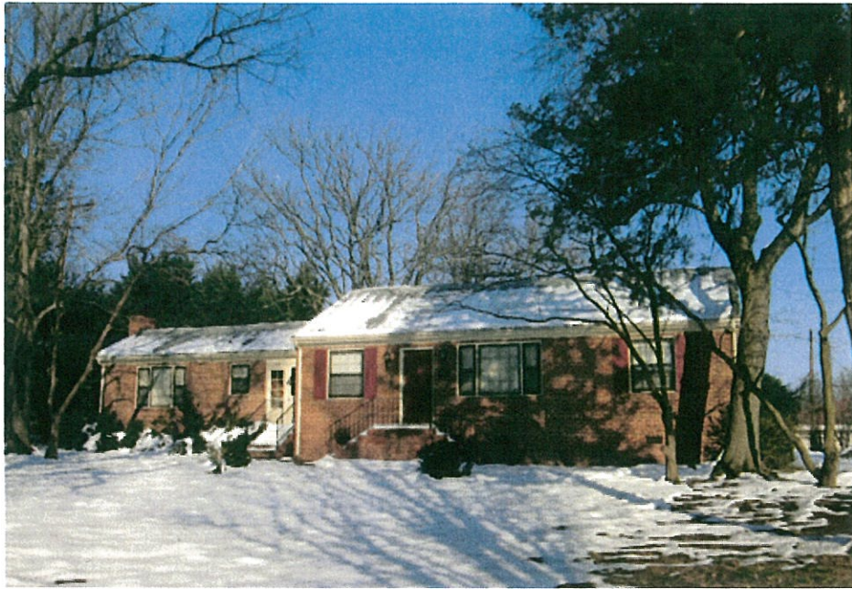
Ranch House at 4217 Hermitage Road (to be demolished)
