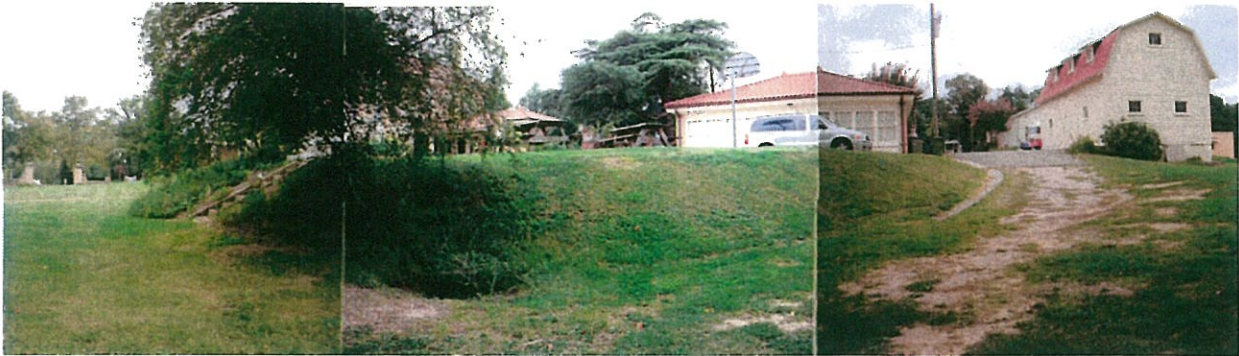
Existing Roadbed and Buildings
