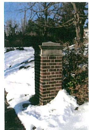
Existing Brick Pier
