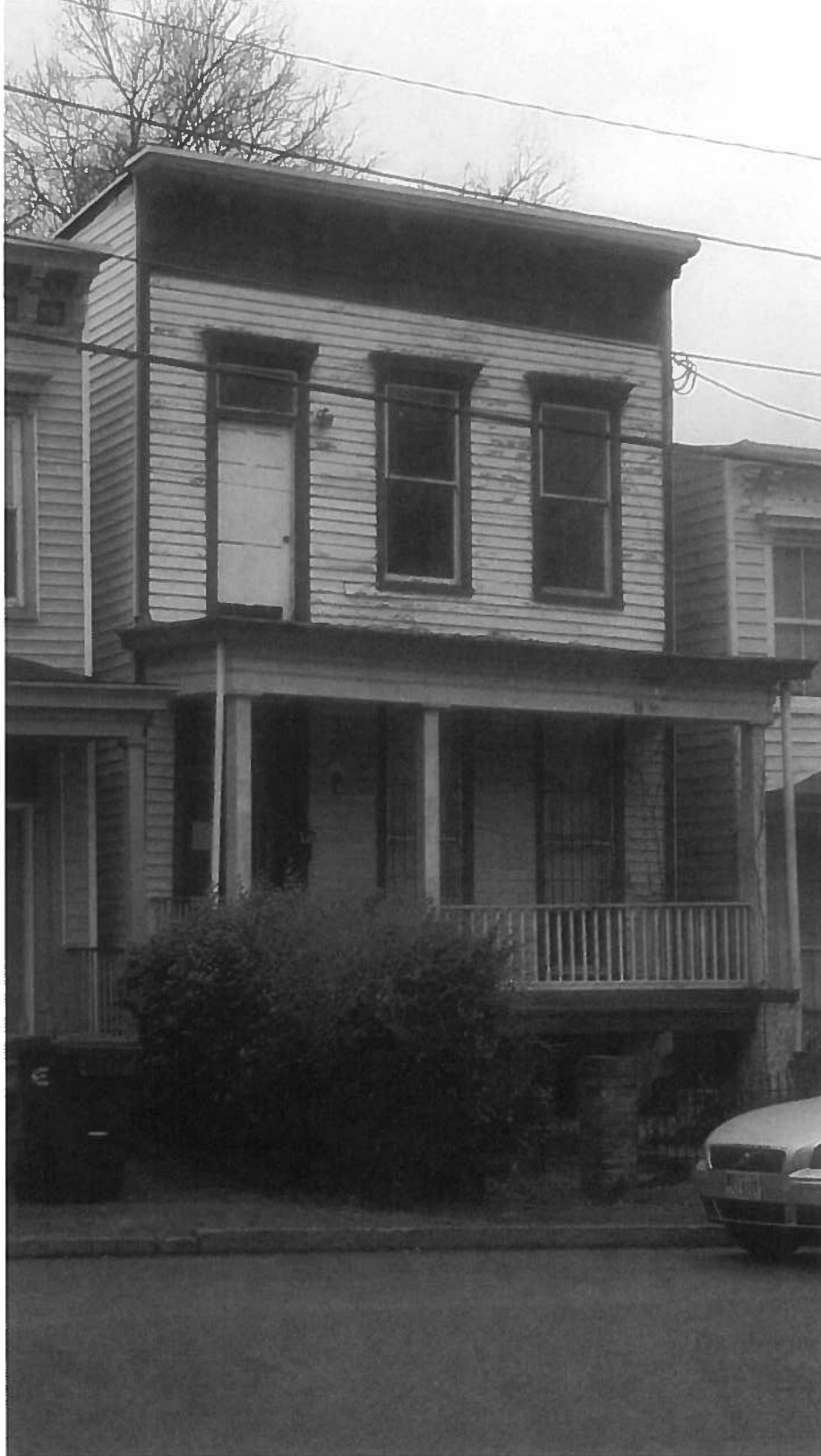
Photo 11. 2109 E. Marshall St with door to original Upper Front Porch
