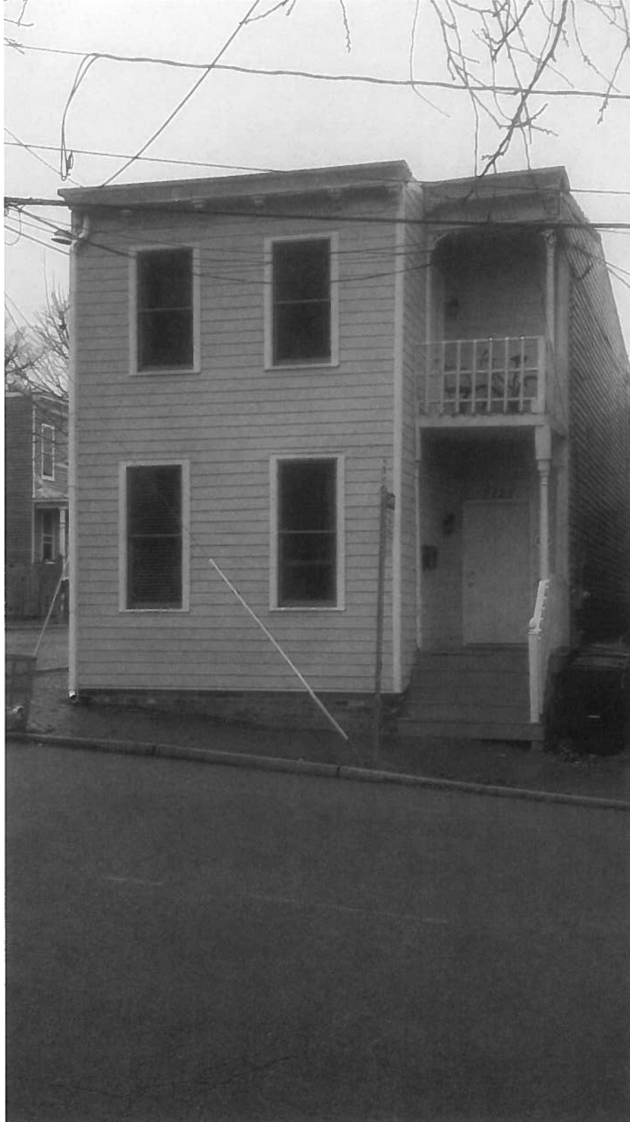
Photo 12. 2123 E. Marshall St with door to original Upper Front Porch
