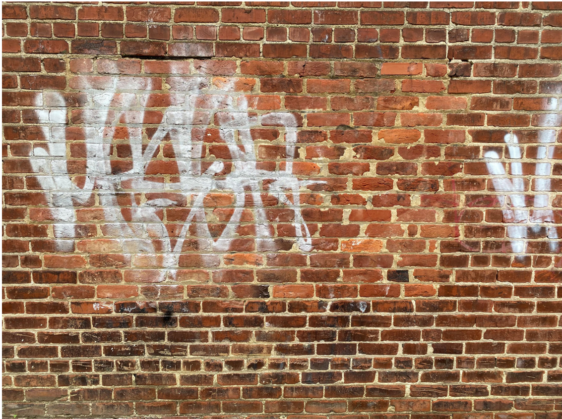
11. Brick infill at alley window opening
