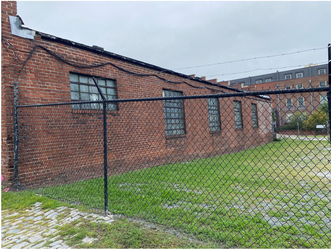
12. Garage west elevation, view from alley
