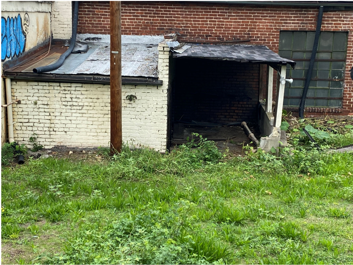
7. Brick boiler room and non-historic shed structure
