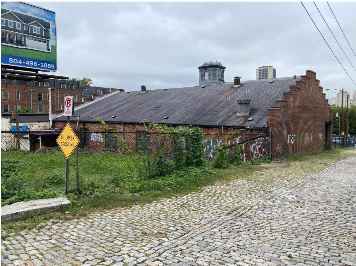
8. East and North elevations, view from alley
