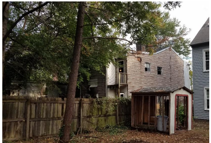
Figure 2. View of east elevation from alley
