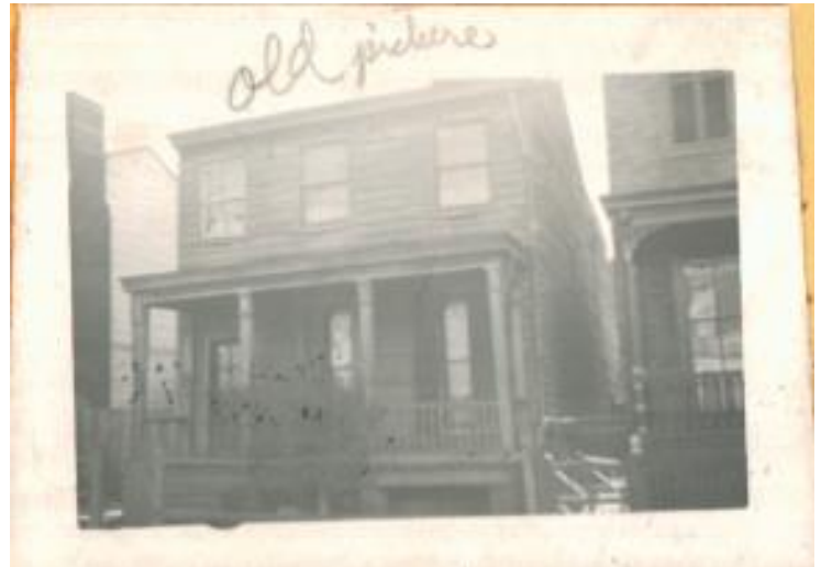
Figure 4. 517 Catherine Street, prior to 1963
