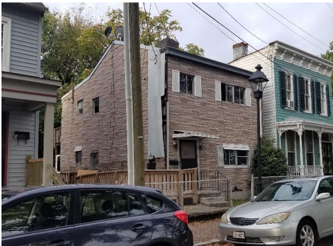
Figure 1. 517 Catherine Street, view from Catherine Street
