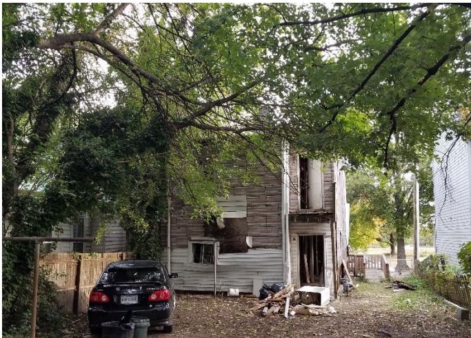
Figure 3. View of south elevation from alley
