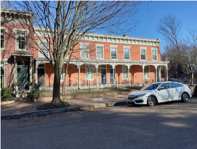
Figure 1. 2218 East Grace Street, façade
