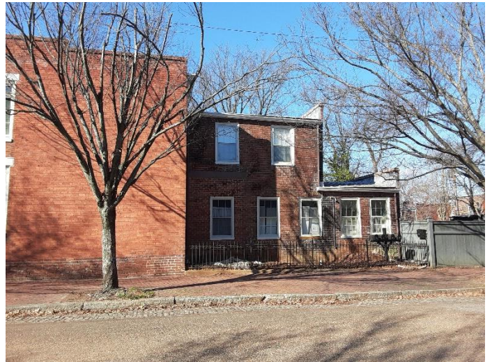
Figure 2. Existing location of mailboxes, east elevation
