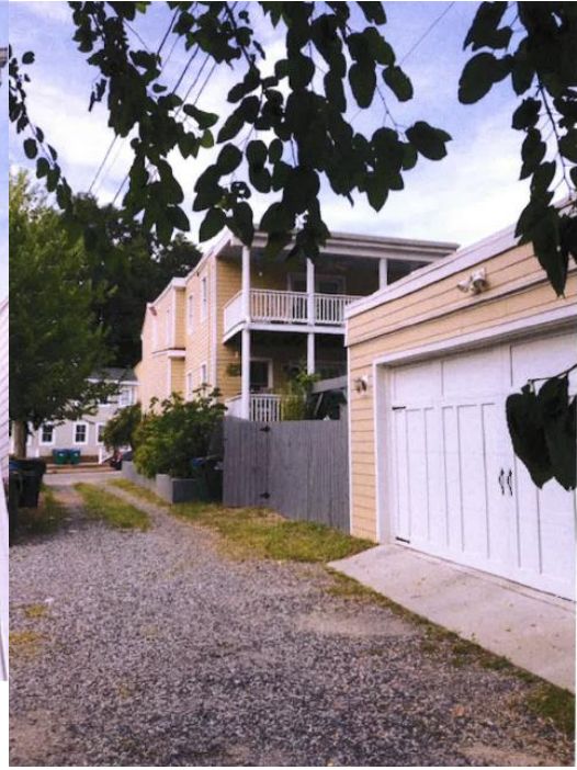
Figure 4. View of 2 nd story rear porch from alley looking NE toward Cedar St.
