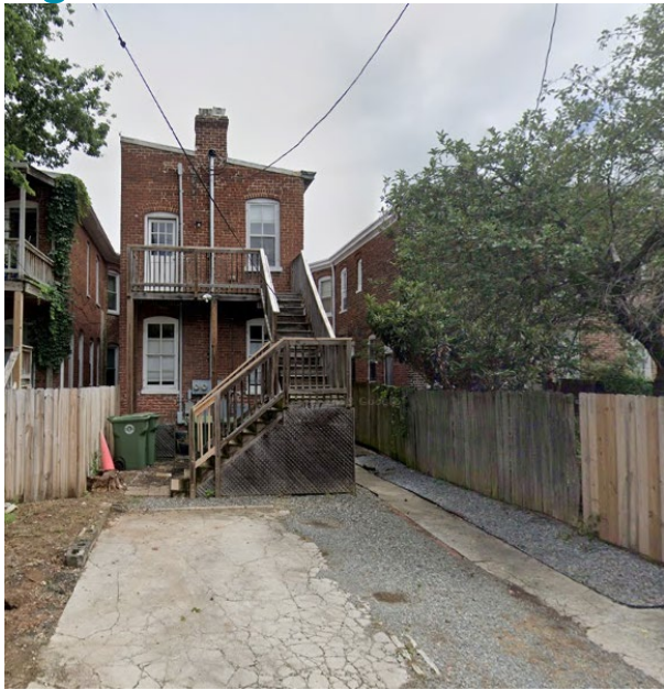
Figure 1. Existing conditions. Rear yard of 1827 West Grace Street. Existing rear deck, fence, and concrete pads visible from alley.
