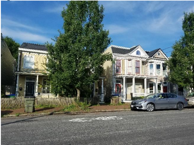
Figure 3. 3013-3015 and 3011 East Marshall Street.
