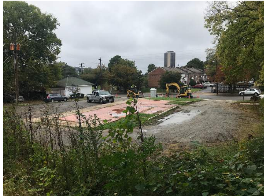
Rear alley with northeast corner in the foreground.
