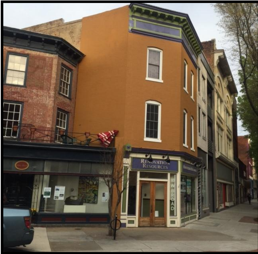
Historic Buildings, Brook Road West-Facing Façade
