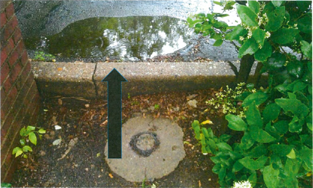
This area fills with water when it rains and turns to ice in the winter.
