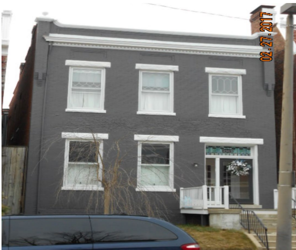
Figure 1. Front Façade, Assessor's Office.
