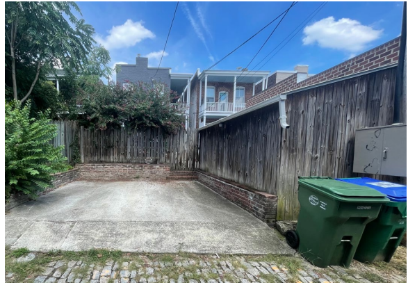
Figure 3. Existing rear parking area, including the 24" brick wall (likely foundation of original garage) and the non-original wooden storage area.
