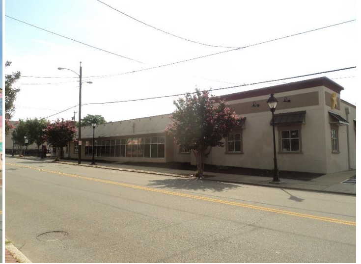
Figure 2. Odd side of North 25th Street, looking northeast, outside of district
