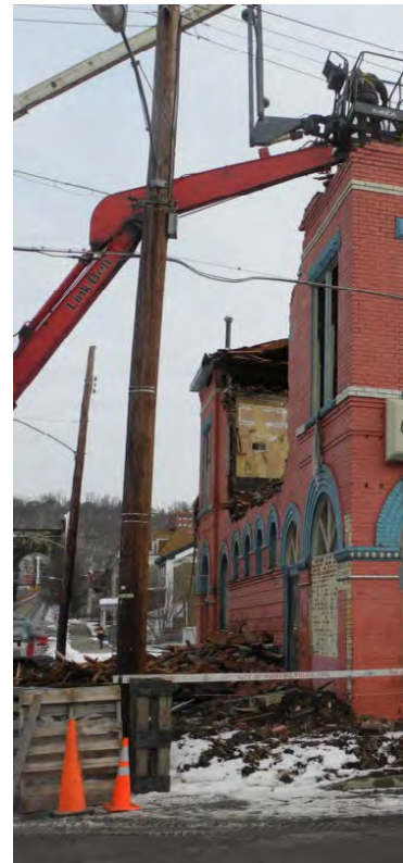
Building Demolition. CPG
