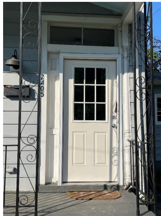
Figure 6. View of the non-historic porch posts.
