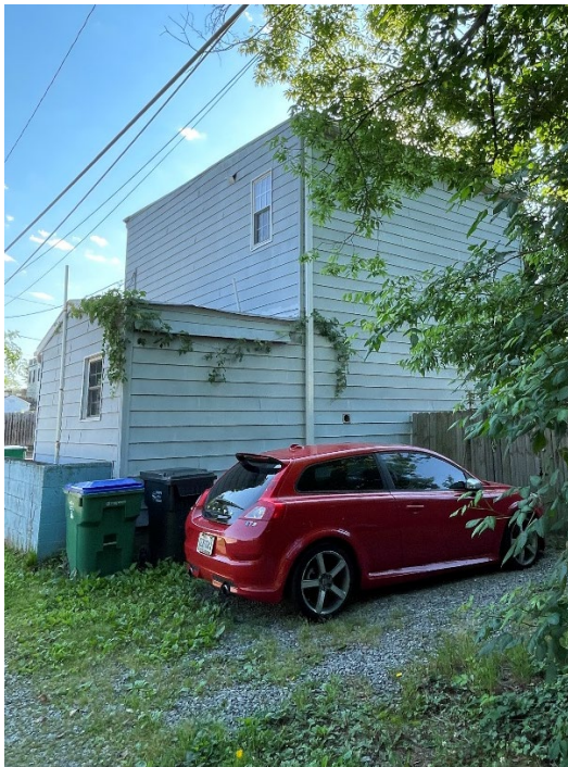
Figure 5. View of the rear, south elevation, from the public alley.
