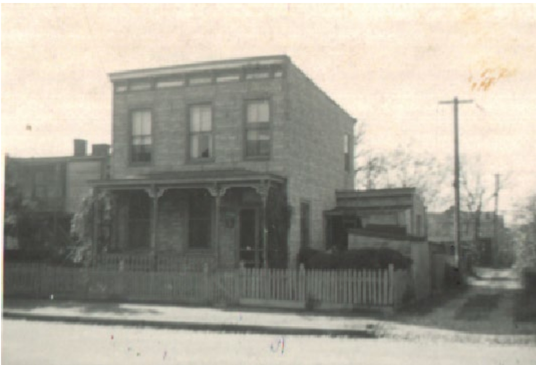
Figure 8. Historic photograph of 2405 O Street with wooden porch posts and potentially shingle siding.
