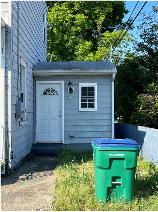
Figure 3. View of the north elevation of the one-story addition.
