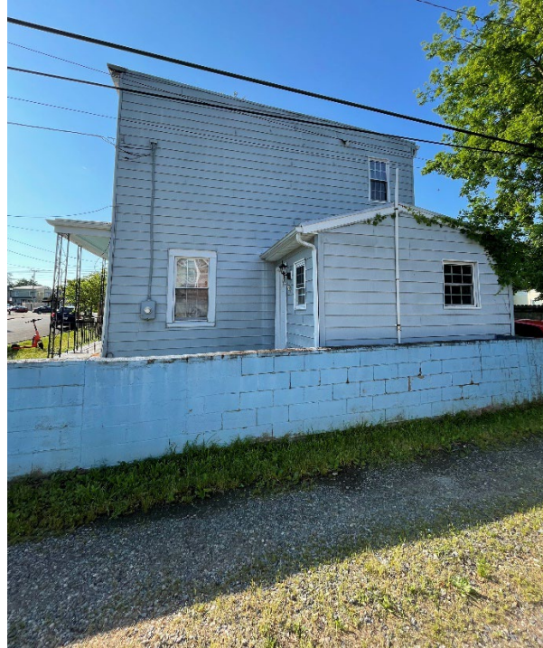
Figure 4. View of the west elevation, from the public alley.
