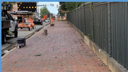
9th Street Improvements
