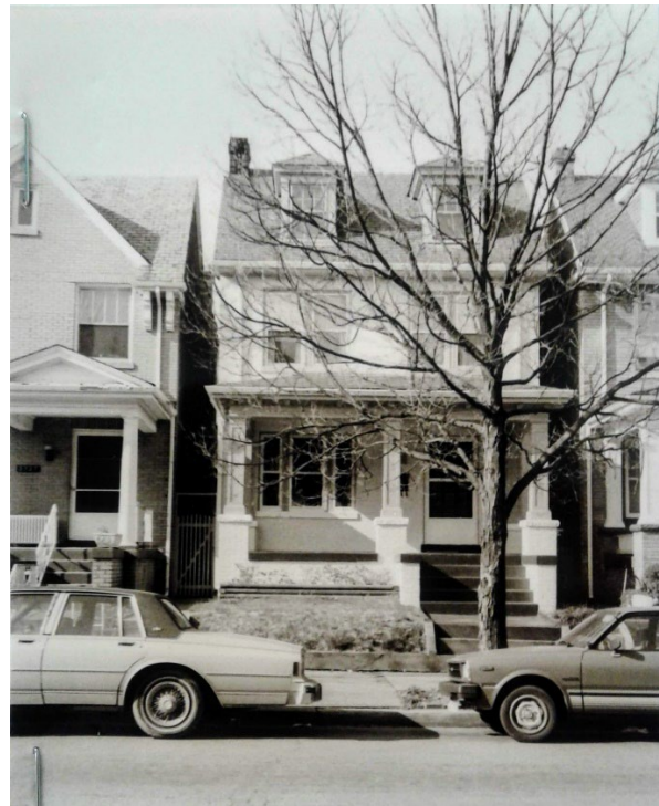
Figure 2. Front elevation of structure 1985.
