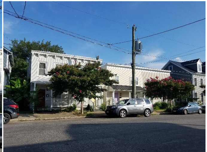
Figure 6. 620-622 North 29th Street.
