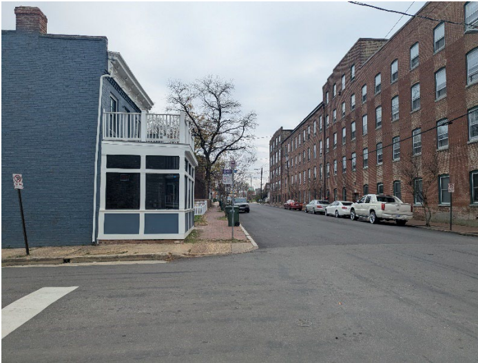
Figure 3. Looking east down Venable Street from subject site.
