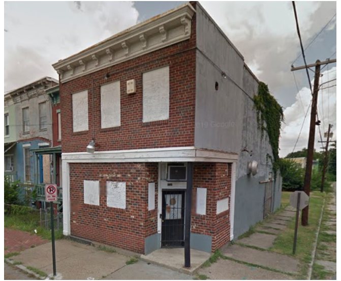
Figure 6. Original mixed-use building located on the Subject Site. Demolished.
