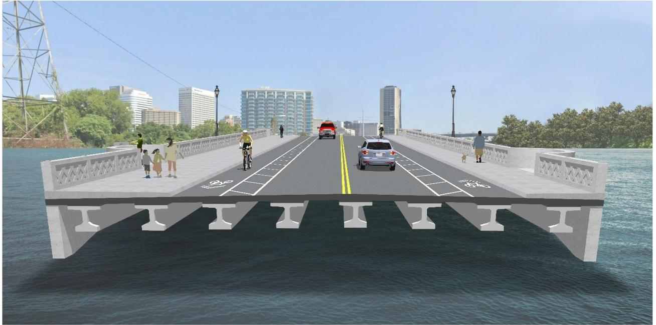
The layout of the bridge will be one vehicle lane and one bike lane in each direction, separated by 4 foot wide spacer markings. The proposed sidewalk is 14 feet on the north side and 8 feet wide on the south side of the bridge. A raised intersection and additional safety features, plus bus pull off lanes, are proposed on Mayo Island.
