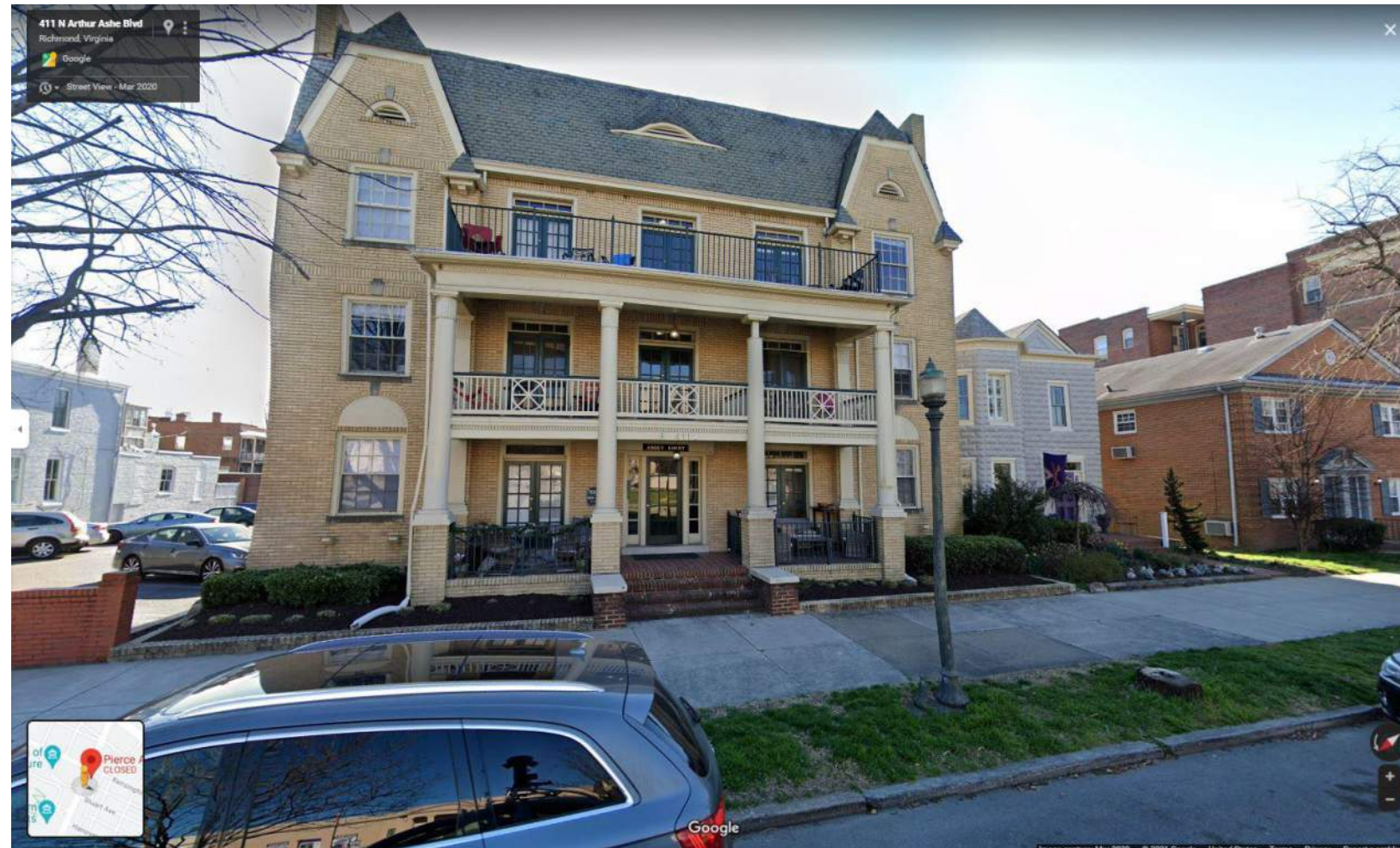
425 ARTHUR ASHE BLVD: RIGHT SIDE OF SITE; FRENCH REVIVAL APARTMENT BUILDING
