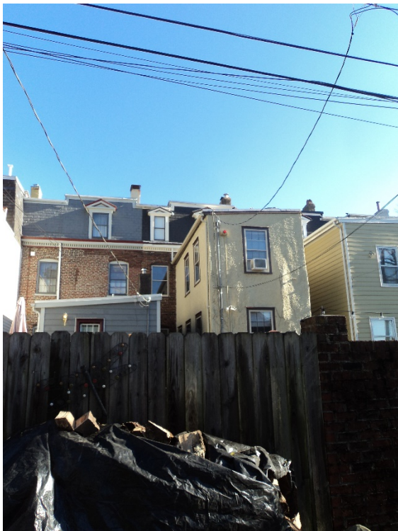
Figure 3. View of main structure from rear.
