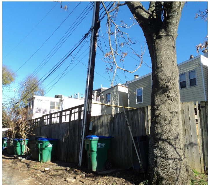
Figure 4. View of structure from rear alley.
