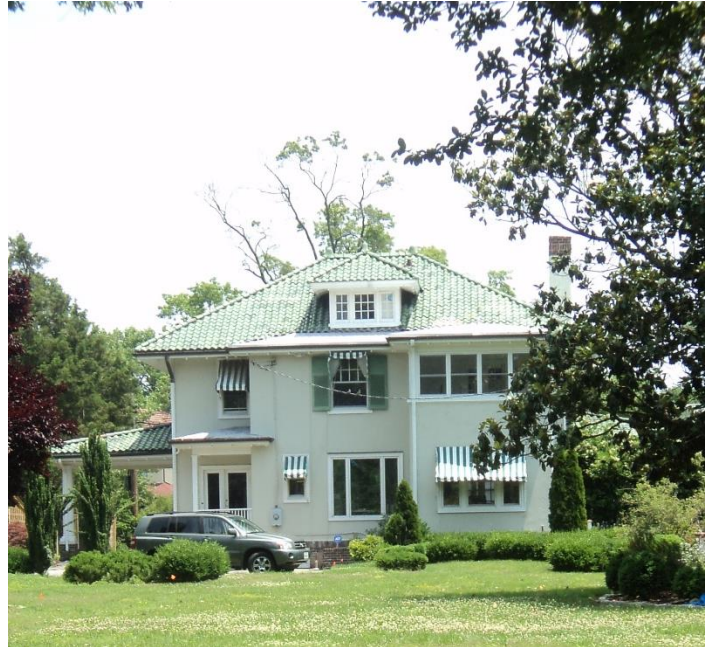
Figure 2. Rear elevation, April 2015
