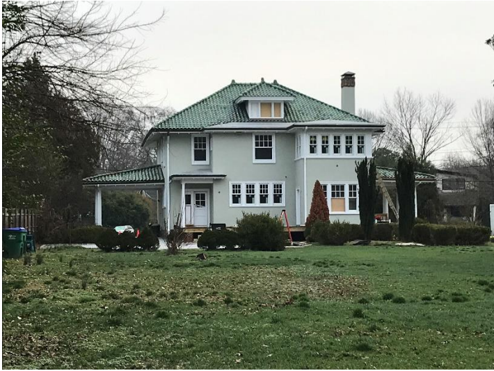
Figure 1. Rear elevation, February 2020
