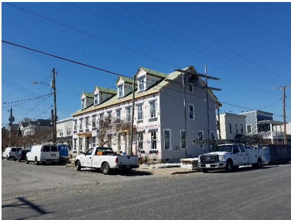
Figure 3. New construction at 2825 M Street.
