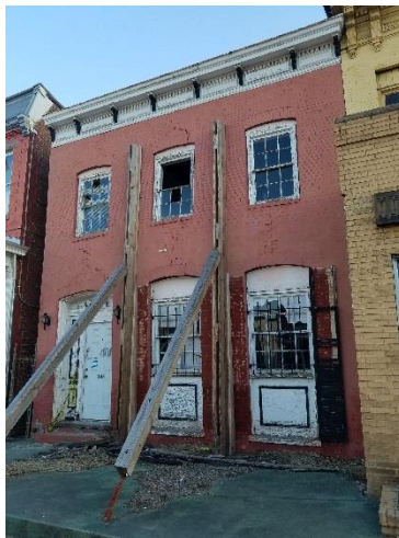
Figure 4. 14 1/2 West Leigh Street, current conditions.
