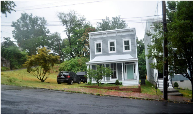
Figure 5. View of 2904 East Franklin Street. The driveway west of 2904 East Franklin Street is the proposed location for 2904.5 East Franklin Street.
