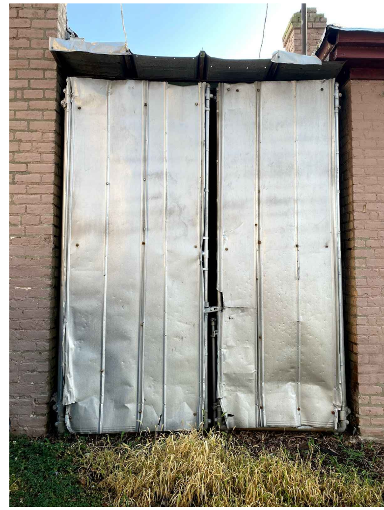
STRUCTURE TO BE DEMOLISHED BETWEEN BUILDINGS 8
