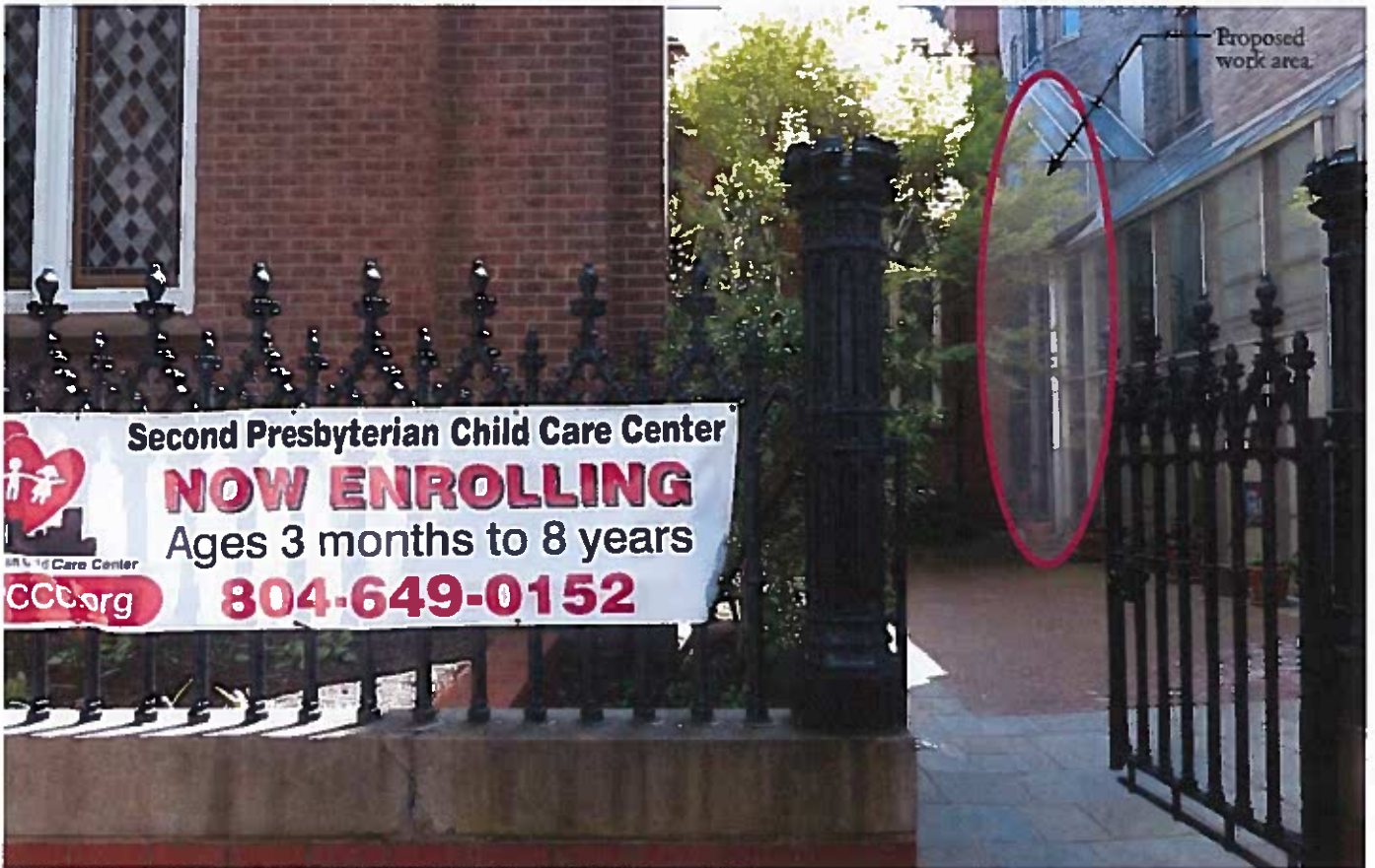
VIEW FROM NORTH FIFTH STREET LOOKING EAST
