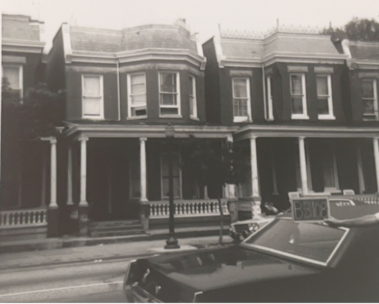
Figure 1. Façade photo ca. 198
