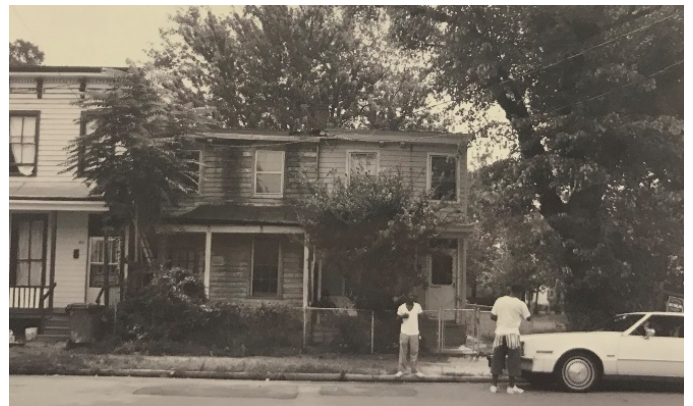
Photograph 2. 807-809 North 24th Street, ca. 1993.
