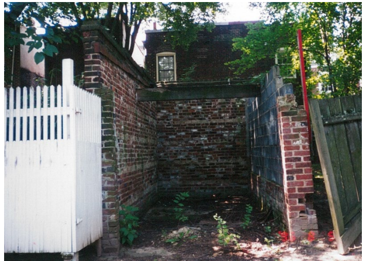
Figure 4. Garage prior to rehabilitation, 1996
