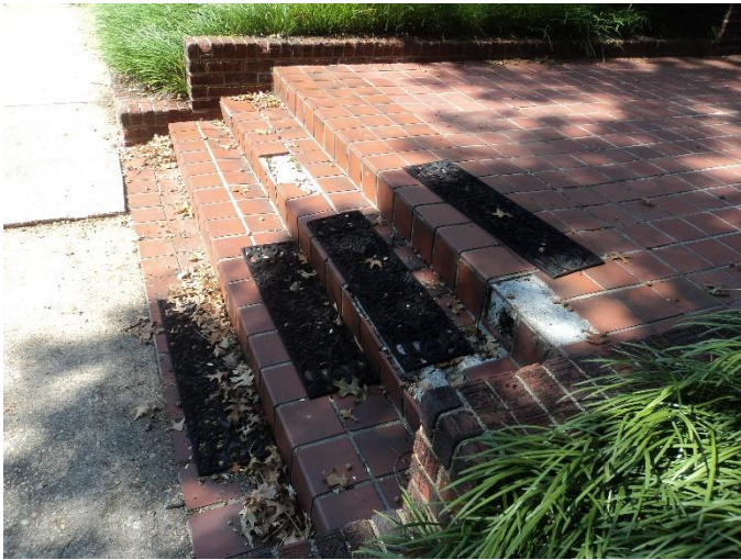
Figure 1. 3006 Monument Avenue, existing condition of front steps
