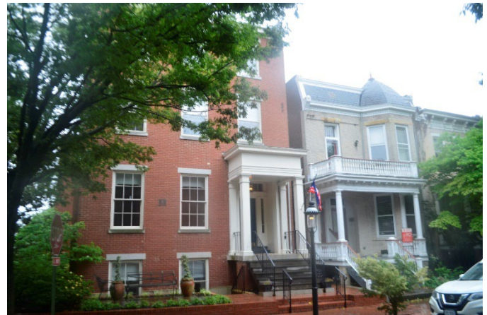
Figure 14. View of 19 and 17 North 29 th Street, located south of the intersection of 29 th and East Franklin Streets. Number 19 was constructed in 1850 while, number 17 dates to 1909. The south section of North 29 th Street, due west of the proposed new building, is an intact historic block. The east side of East Franklin Street has greatly changed over the past several decades with only one historic building visibly intact.
