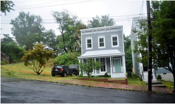
Figure 5. View of 2904 East Franklin Street. The driveway west of 2904 East Franklin Street is the proposed location for 2904.5 East Franklin Street.
