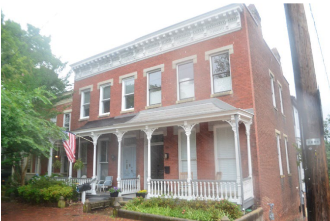
Figure 13. View of 101 North 29 th Street, which was constructed in 1891. This house is on the northwest side of the intersection of 29 th and Franklin Streets. The south side of this house is along East Franklin Street. The rear of the house has had several additions in recent years and is due west of 2904 East Franklin Street.
