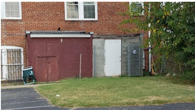
Figure 3. Existing sheds to be removed.
