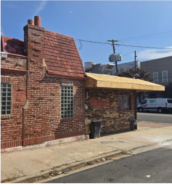
Figure 2. 1000 N 25 th Street – Repair to canopy underway and new glass block windows installed.
