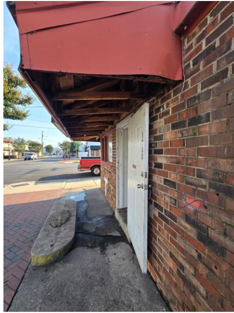
Figure 2. 1000 N 25 th Street – View of façade along N. 25 th Street.
