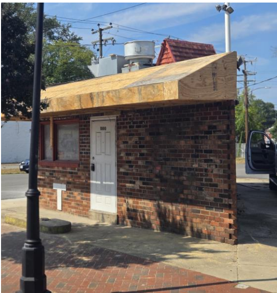
Figure 3. 1000 N 25 th Street – Repair to canopy underway.
