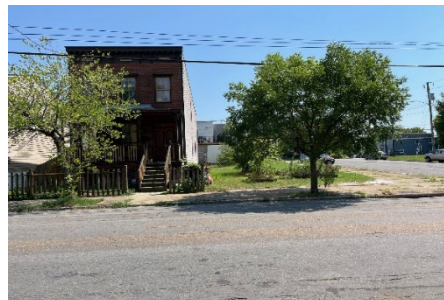
Figure 6. Southeast corner of Venable Street and N. 22 nd Street.
