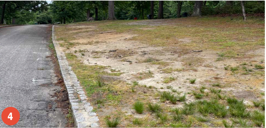
4 Erosion on Site
