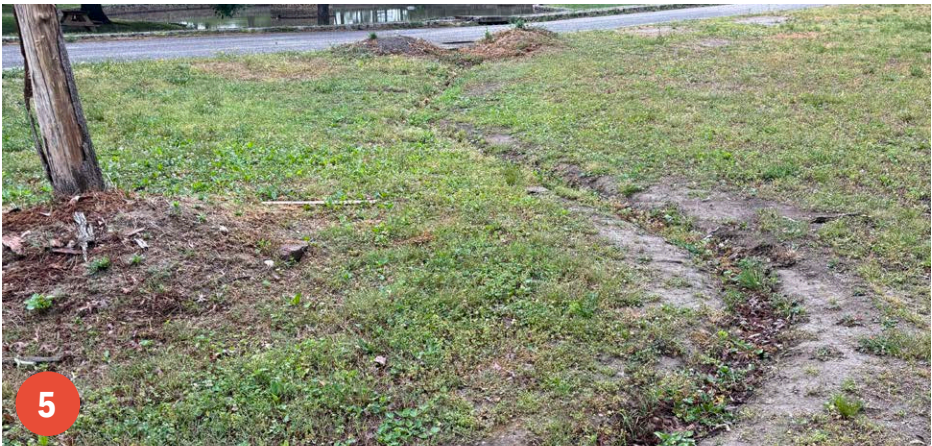
5 Erosion on Site
