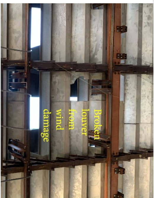
Example of broken louver from wind damage that
