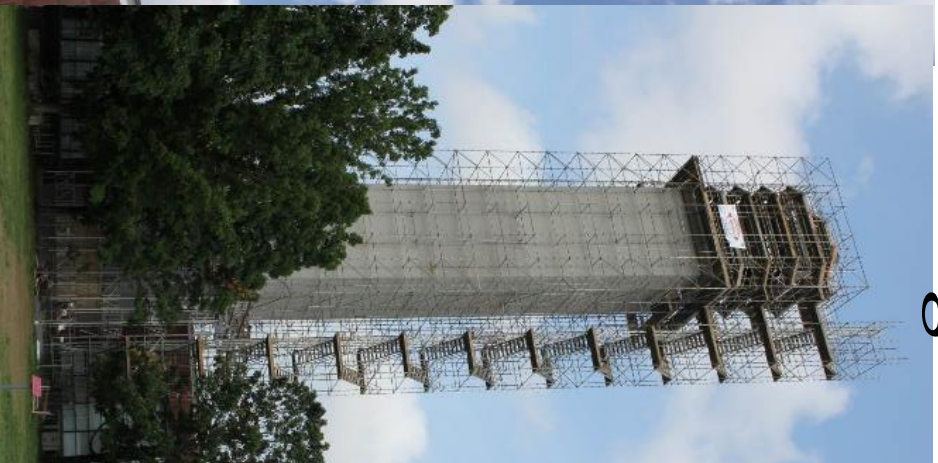
The Belgian Pavilion, Tower Structural Repairs Richmond, Virginia Photograph, 24 May 2012
