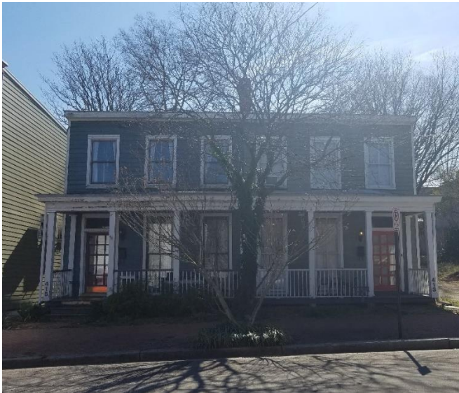
Figure 7. 413-415 North 22nd Street.
