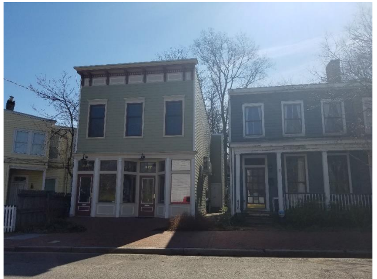
Figure 8. 417 North 22nd Street.
