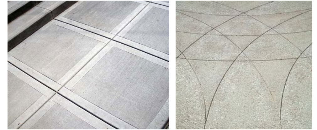
CONCRETE SCORING PATTERN FOR SIDEWALK
