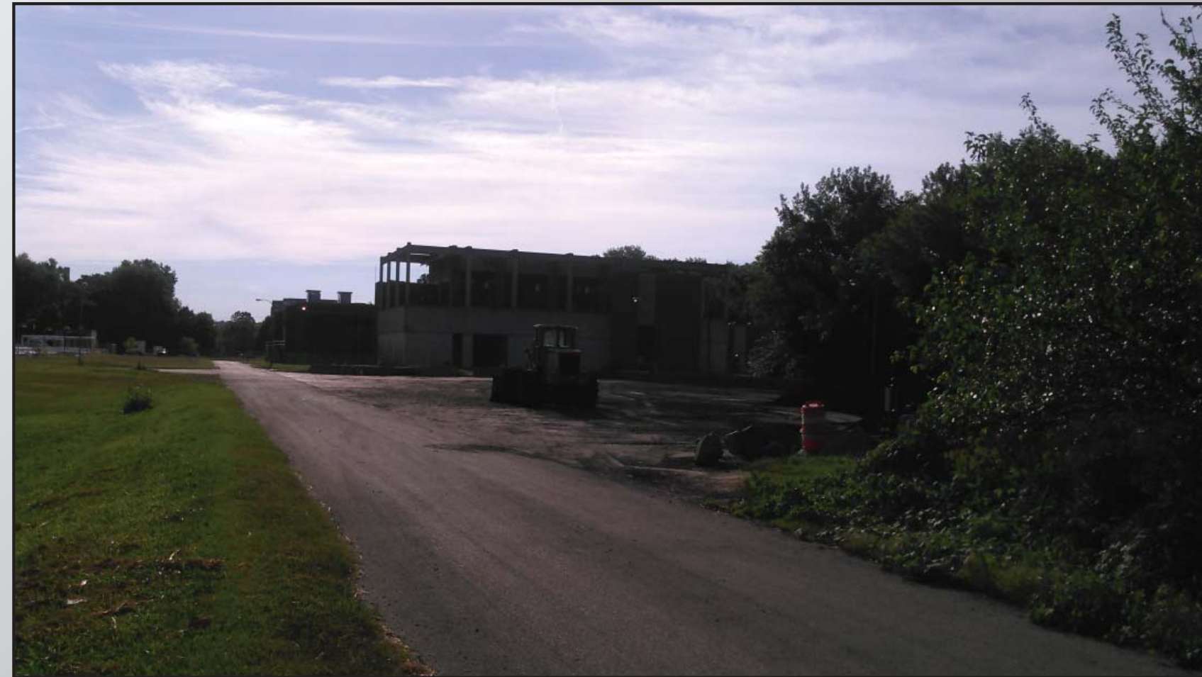
Existing Biosolids Storage Pad Facing East
