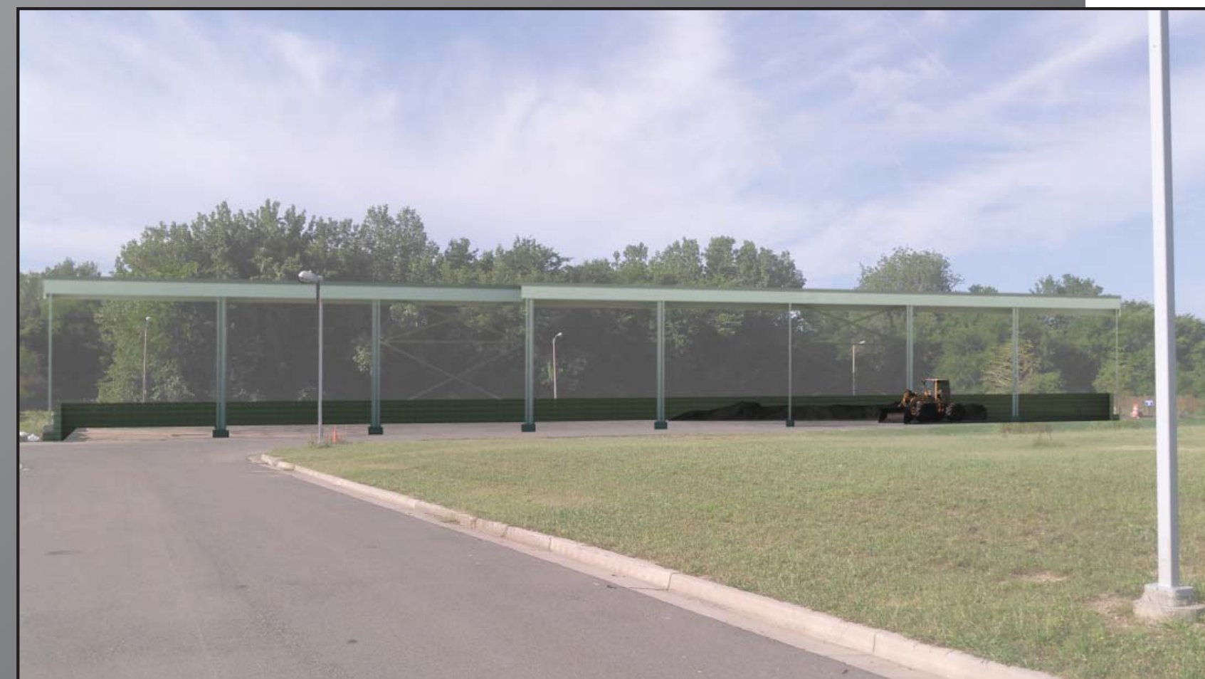
Proposed Biosolids Storage Pad Facing South
