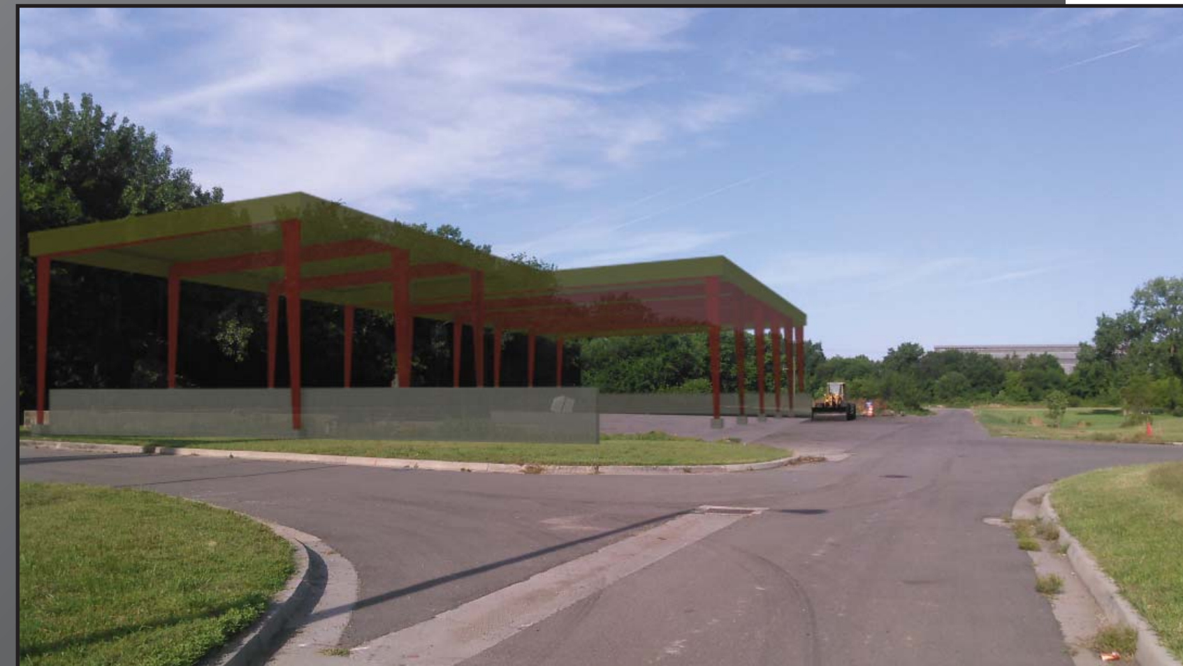
Proposed Biosolids Storage Pad Facing West
