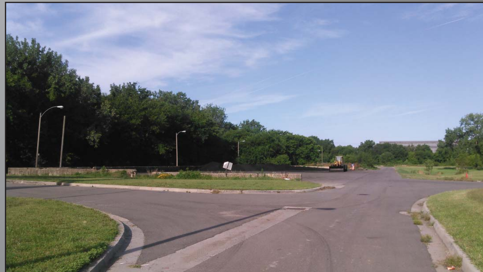
Existing Biosolids Storage Pad Facing West
